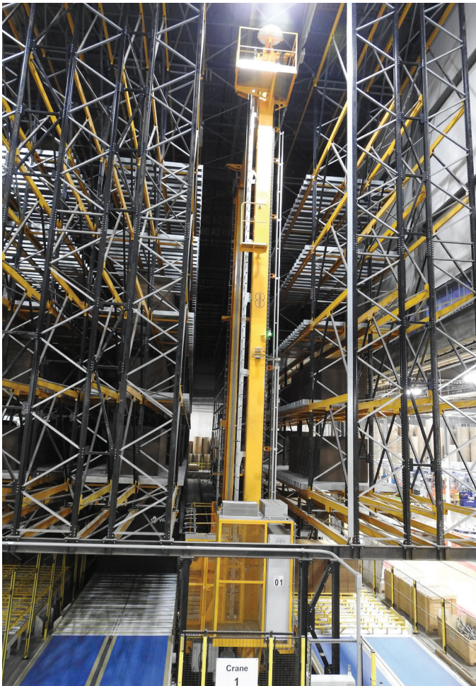
WSA USA and partners installed a cutting edge rack system.
